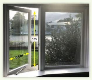
multiply these measurements to reach a total openable area of windows, doors and skylights. Using the image above, the calculation would be 1 x 0.6
